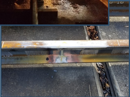
Two rail sticks joined after flashbutt welding
