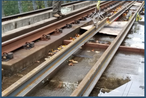
Rails placed and aligned for flashbutt welding
