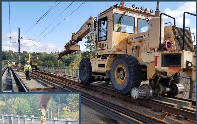
Track Maintainers removing old rail from the line and threading the new
